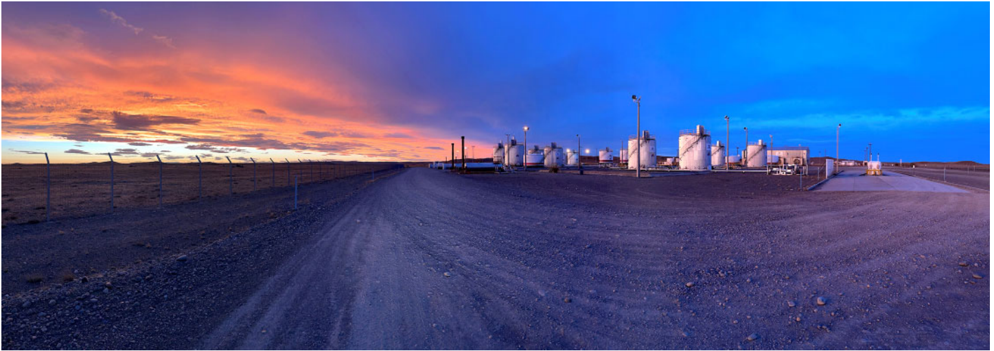
Oilfield treatment plant
