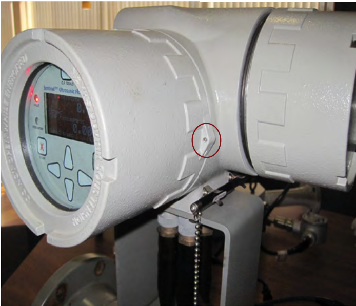
Figure 34: Front cover screwed
