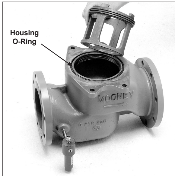
Figure 7b - 6" FlowMax: remove cage & inspect housing o-ring
