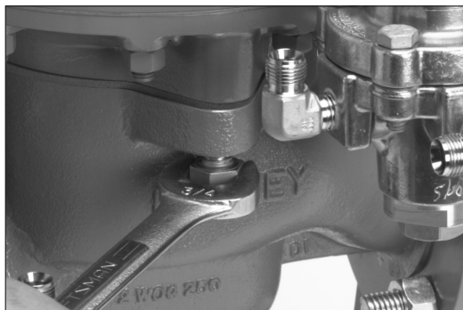
Figure 43 - Tightening the body cap screws
