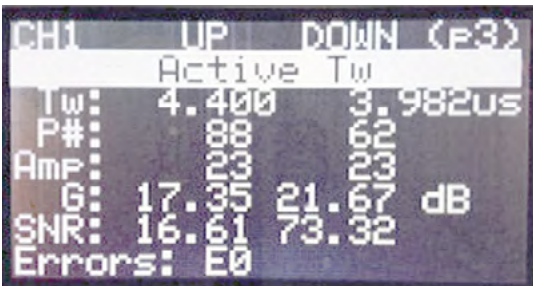
Figure 60: Flow info - active Tw CH1
