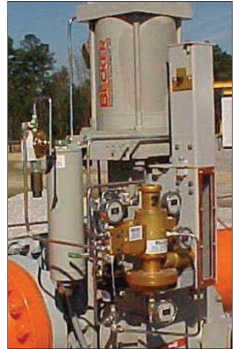
Figure 8 – HPP-4 with VB-250 Volume Boosters
