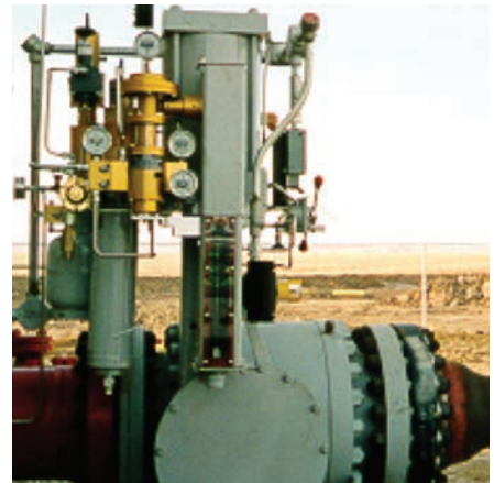
Figure 9 – Becker HPP-3 Positioner with RPDA Actuator
