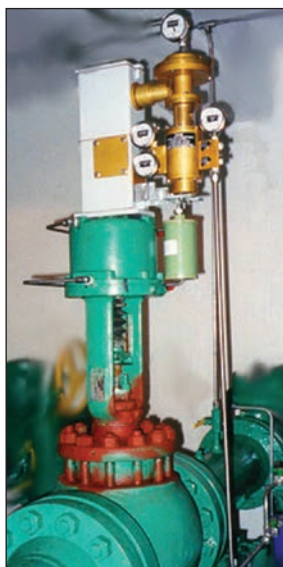
Figure 7 - Becker Model HPP-3 Positioner Retrofit to Fisher Type 470 Actuator.
