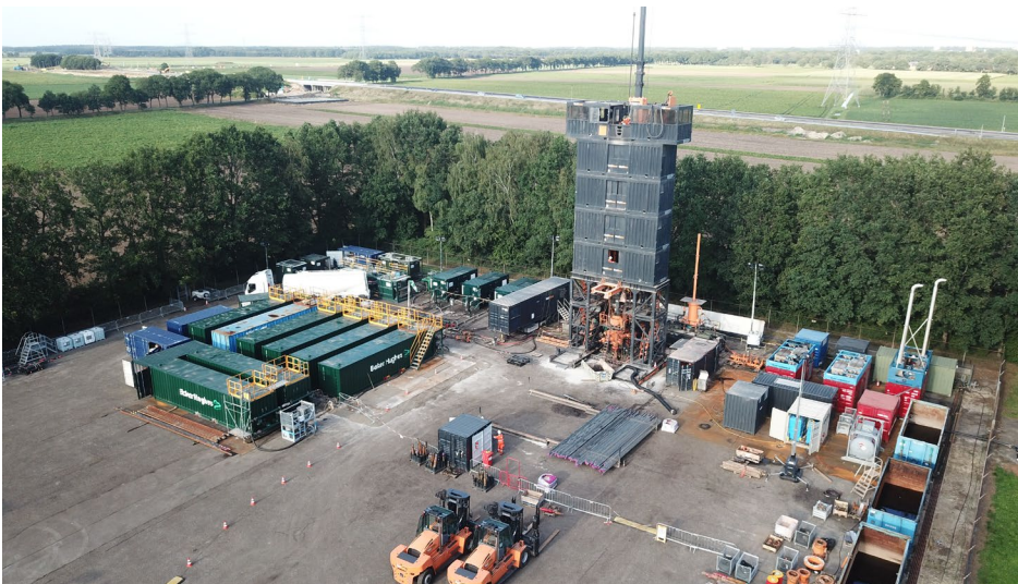
This is the first fully integrated well abandonment approach which included a 100% electric P&A unit that significantly reduced CO 2 emissions, smell, and noise contour.
