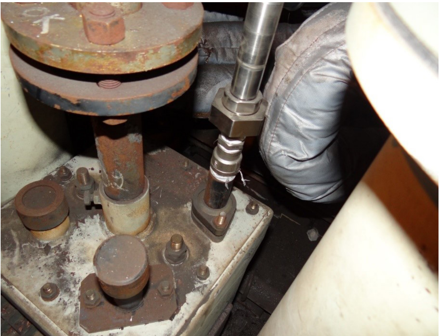
Figure 3 – FTD 325 Hot end connected to the sensor position of the burner
